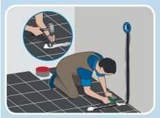
Cut a groove into the floor and wall 10mm deep and 10mm wide for the floor sensor and tube. The tube allows for easy removal of the floor sensor if required.
