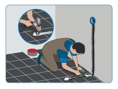
3) Cut out a wall groove and fix cable ducts and connection box. Chisel off a groove for the sensor conduit and cold cable. Fix the sensor conduit e.g. with a glue gun.
