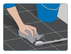
4) Clean the sub floor in order to protect the cable during installation and to ensure the maximum adhesion of the mat.
