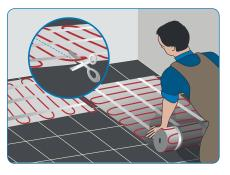
5) Roll out the mat. Cut and turn the mat when meeting walls or obstacles. DO NOT CUT THE CABLE. Min 2 cm between any two cable lines.
