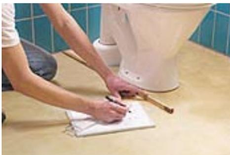
**2.** Mark the positions of the floor fitting objects that will be installed once the floor is finished, so when laying the floor these can be avoided.
