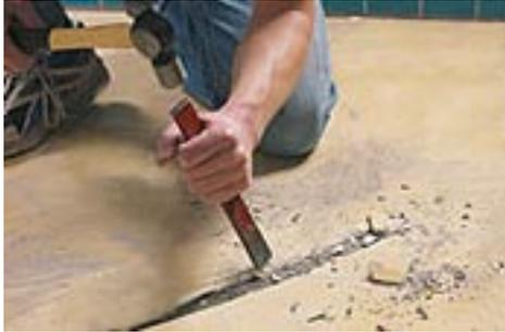
positioned such that it lays between two heating wires and not across them and not above heating pipes below the floor. The end of the tubing in the floor is sealed with tape to prevent adhesive entering the tube.
