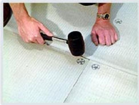
Aquapanel Thermal is a lightweight insulated tile backing board developed specifically for use with tiled floors. It consists of a Polyfoam core with glass fibre reinforced polymer-modified cement faces.
