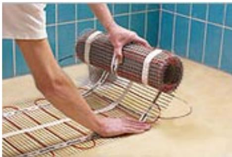
tiling, this may include cleaning and removing all loose particles, removing any sharp protrusions that may cause damage to the heating wire, priming the floor surface bracing a timber floor with WBP ply-for professional guidance refer to your adhesive manufacturers recommendations.
