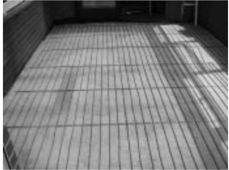
5. A piece of flexible tubing is laid in the floor to house the floor sensor, this should be laid 50-60cm across the floor between a heating cable loop.
